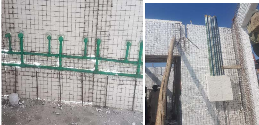
Figure 07: Installation of utilities before concreting
