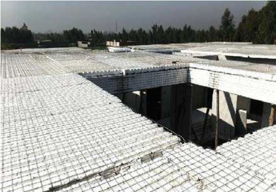
Figure 06: Placed Slab panels on wall panels
