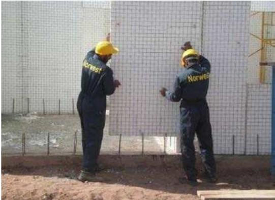
Figure 05 : Placing panels in dowels
