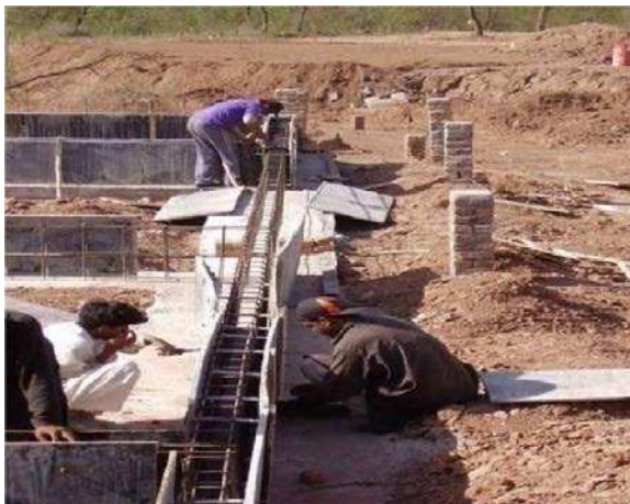
Figure 02: Making of foundation
