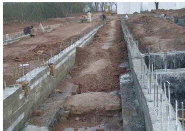
Figure 03: Leaving dowels in foundation
