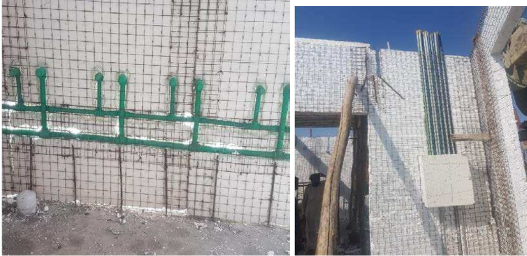
Figure 07: Installation of utilities before concreting
