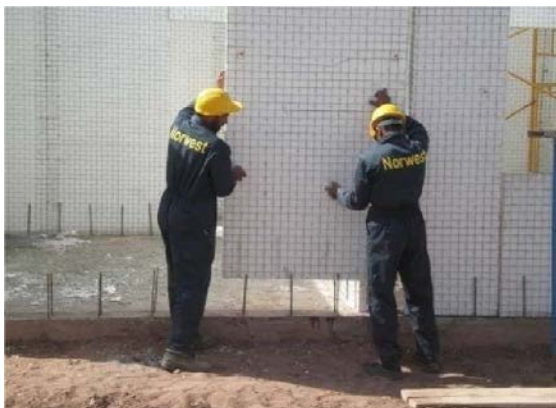
Figure 05 : Placing panels in dowels
