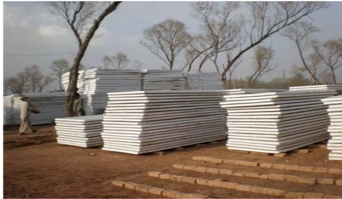
Figure 04: Transportation of panel to site
