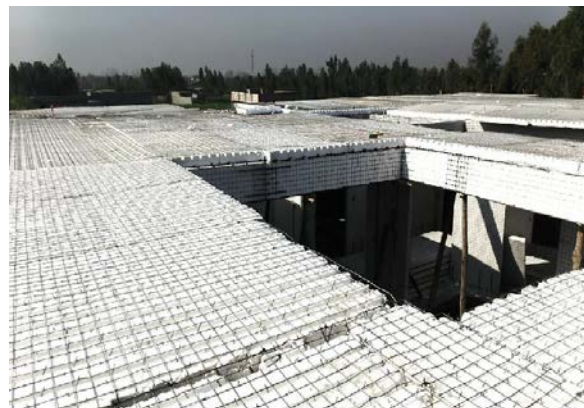
Figure 06: Placed Slab panels on wall panels
