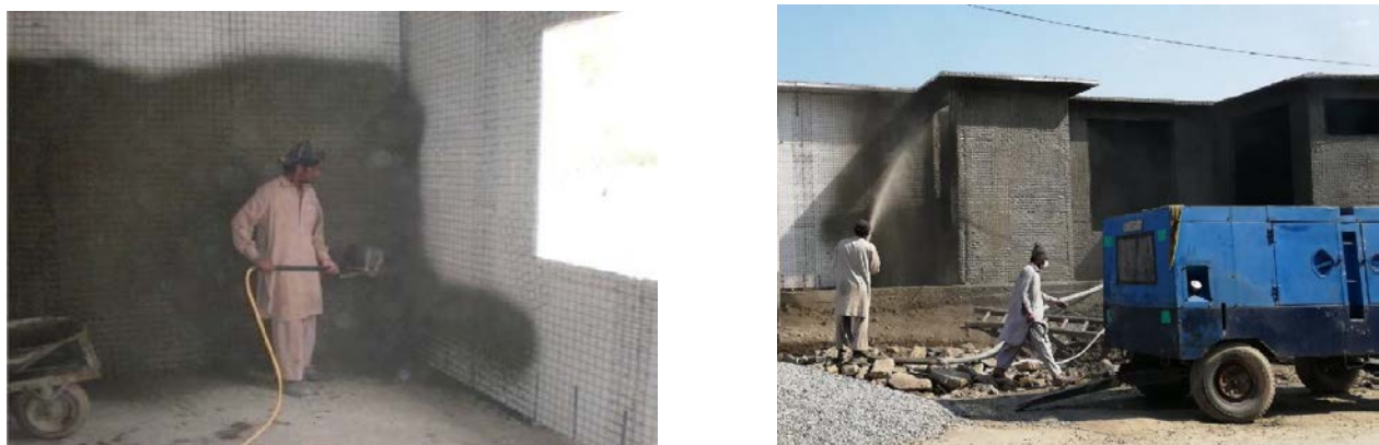
Figure 08: Applying Concrete
