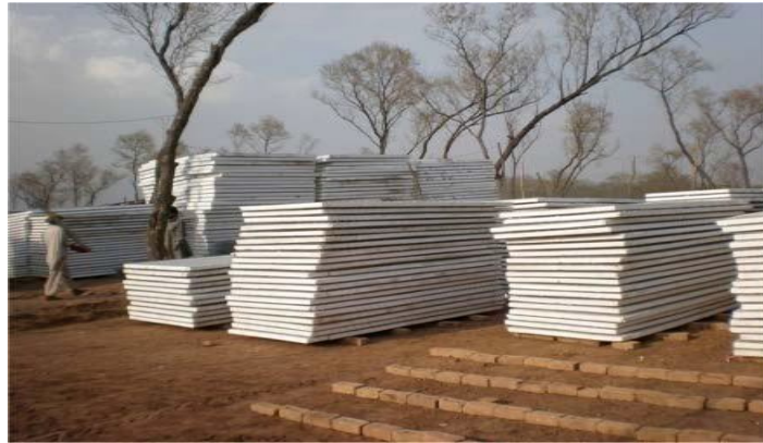
Figure 04: Transportation of panel to site
