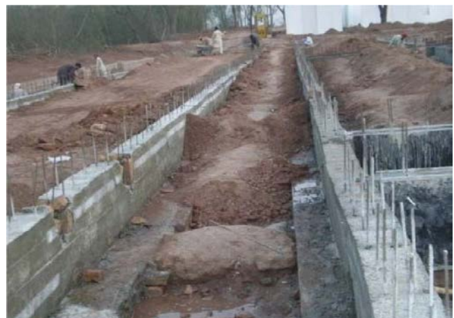
Figure 03: Leaving dowels in foundation
