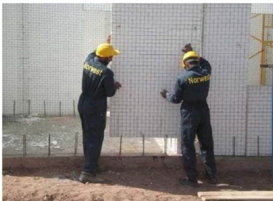
Figure 05 : Placing panels in dowels
