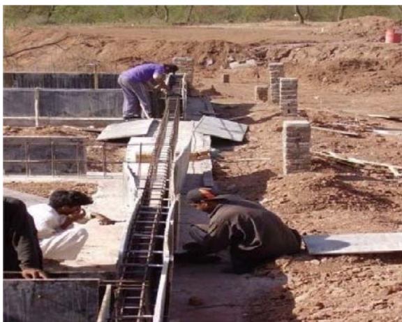
Figure 02: Making of foundation
